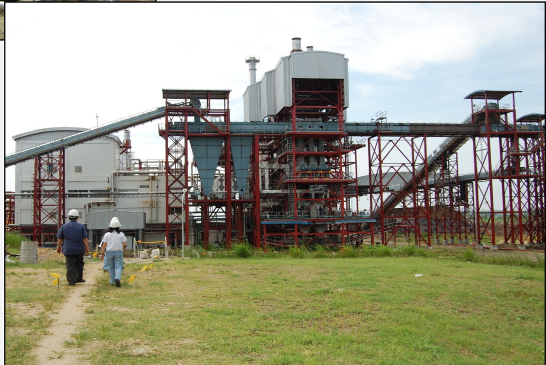
Co-generation Plant (SCBI) ➤
